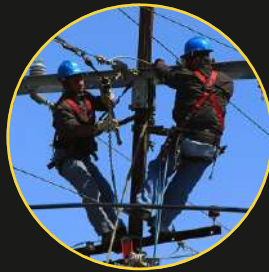
Work at height
